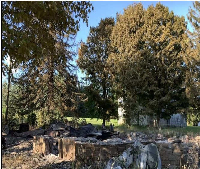
L: Remnants of foundation are all that remain.
